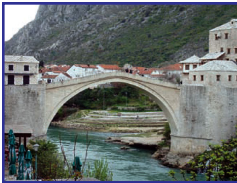
Mostar Bridge, Mostar
